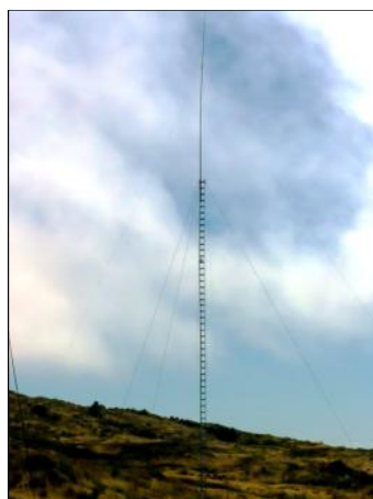
Our second 160 meter antenna was 28 meters tall and top loaded, and used every day, except the first.
