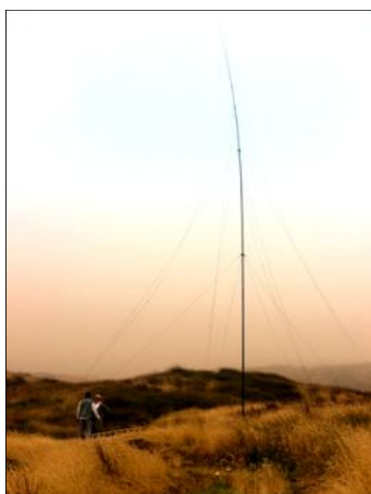
Our first 160 meter antenna was a top-loaded 18-meter tall push-up mast.
