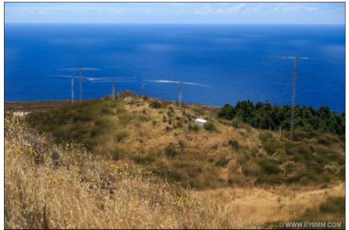
Antennas at the Antonelli site.
